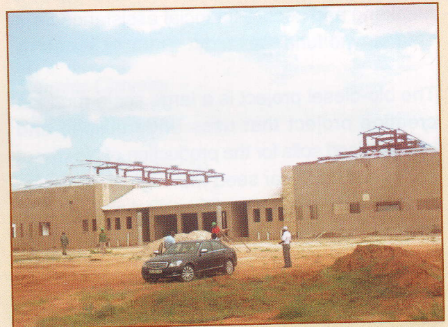
Construction is ongoing at the project site
