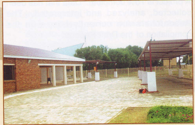
A picture of the complete Car Wash Project situated at unit 7 in Mmabatho
